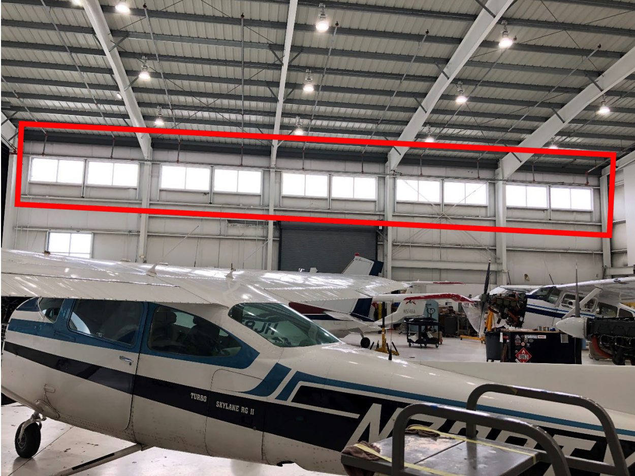
Interior, Looking South
