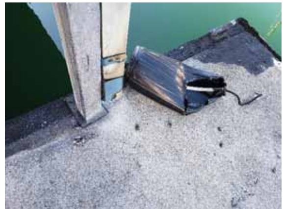
Figure 4 - Outer Roof Column Foundation
