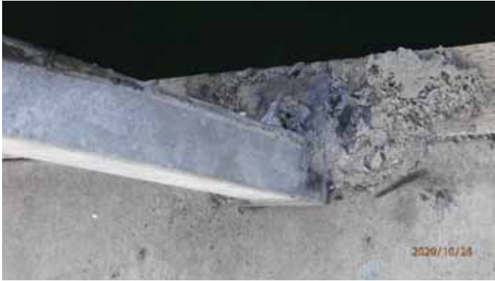
Figure 2 - Inner Roof Column Foundation
