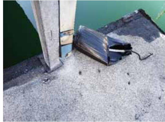
Figure 3 - Outer Roof Column Foundation
