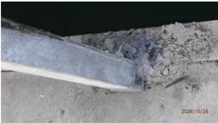
Figure 3 - Inner Roof Column Foundation
