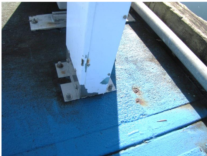
Photo E2.3-8: Powercenter with new angle brackets
