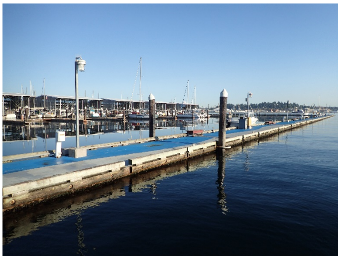
Photo S2.2-3: Overall of Breakwater Float (Looking North)
