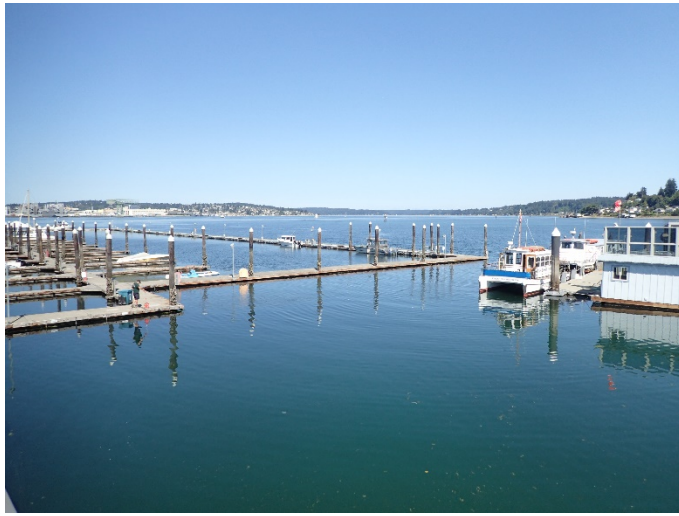
Photo S2.2-1: Overall of East Breakwater (Looking Northeast)
