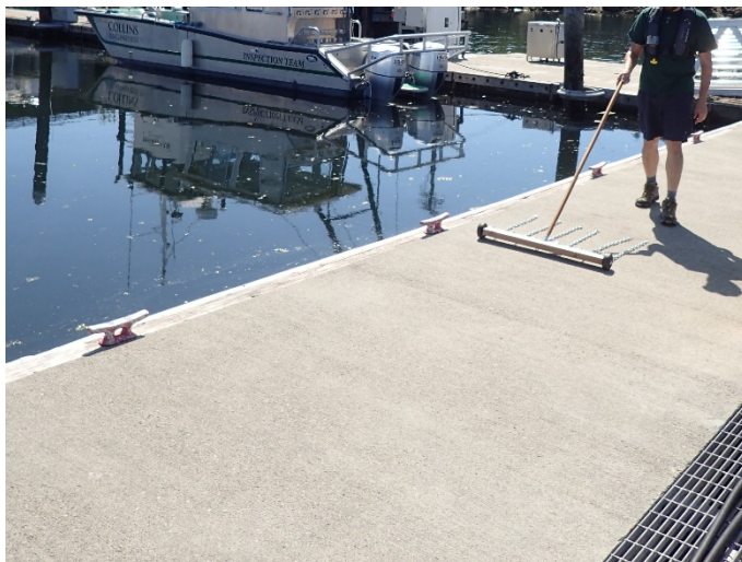
Photo S2.4-8: Typical Condition of Fuel and Breakwater Float Modules
