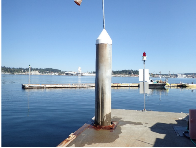
Photo S2.4-4: Typical Guide Pile Condition
