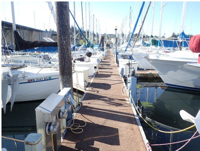
Photo S2.1-2: Overall of A-Dock (Looking North)
