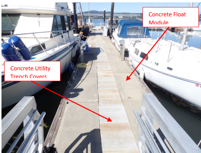
Photo S2.4-3: Overall of Service Float (Looking West)
