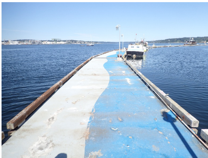
Photo S2.3-3: Overall of North Breakwater (West End, Looking East)
