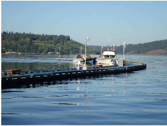
Photo S2.3-1: Overall of North Breakwater (West End, Looking Southwest)
