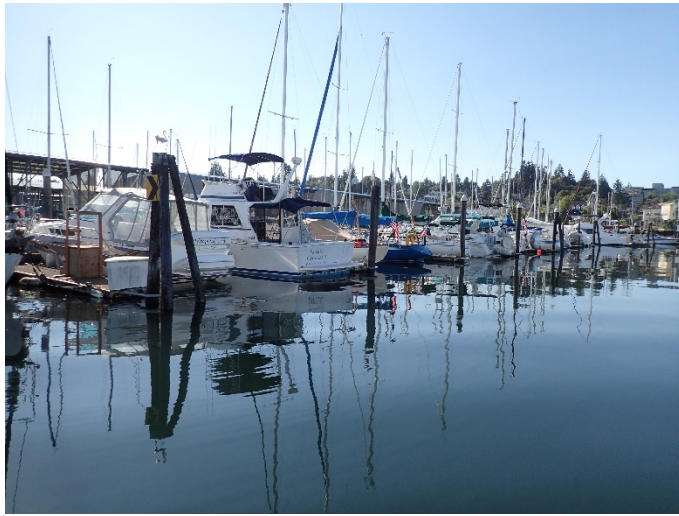
Photo S2.1-1: Overall of A-Dock (Looking Southeast)
