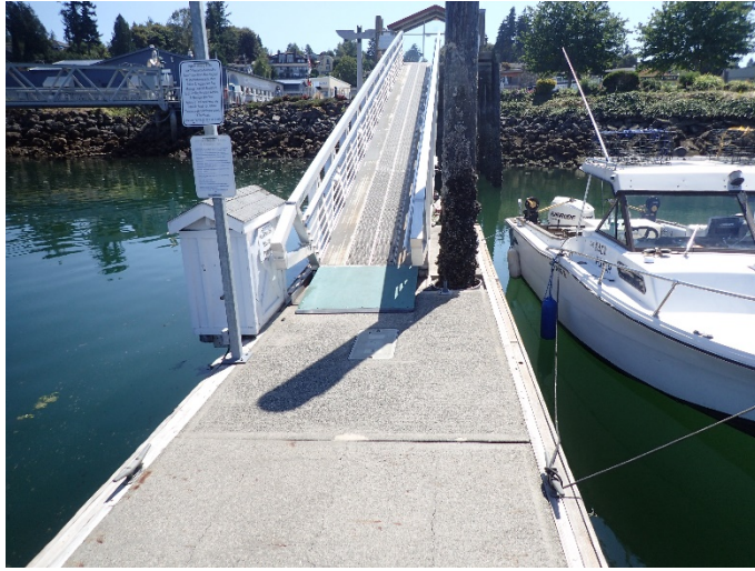
Photo S2.2-4: Overall of Gangway (Looking South)
