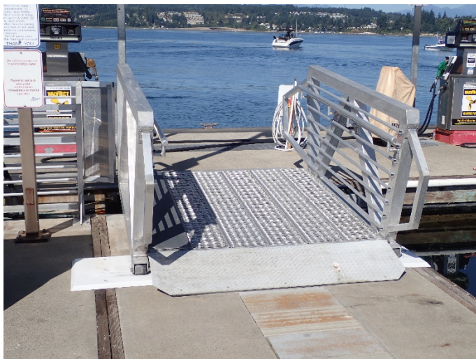
Photo S2.4-5: Condition of Transition Gangway
