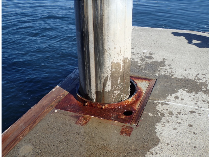
Photo S2.4-13: Typical Guide Pile Assembly Condition
