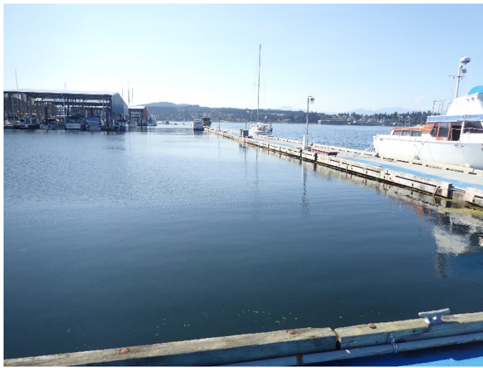
Photo S2.3-2: Overall of North Breakwater (East End, Looking West)
